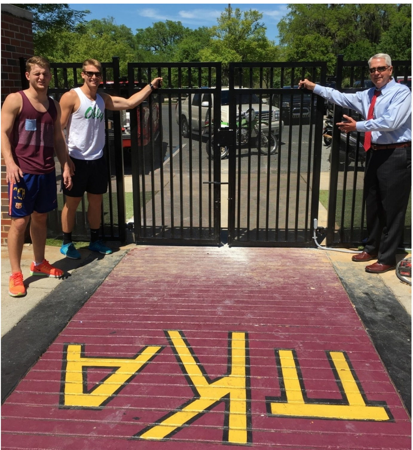
The contractors have just finished installation of the new courtyard gate!" Jimmy Keen
