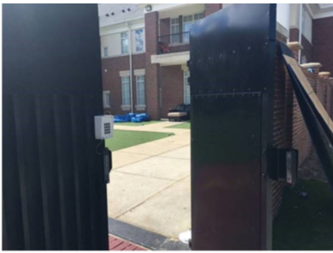
Here are exterior and interior views of the new magnetic-lock back gate entry into the courtyard.
